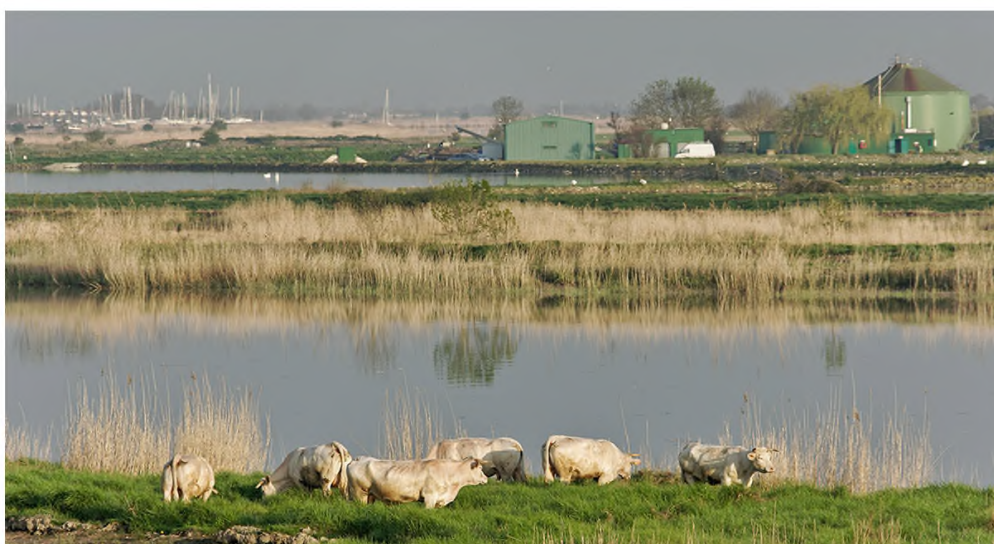
Station de lagunage - Ph. DREAL
