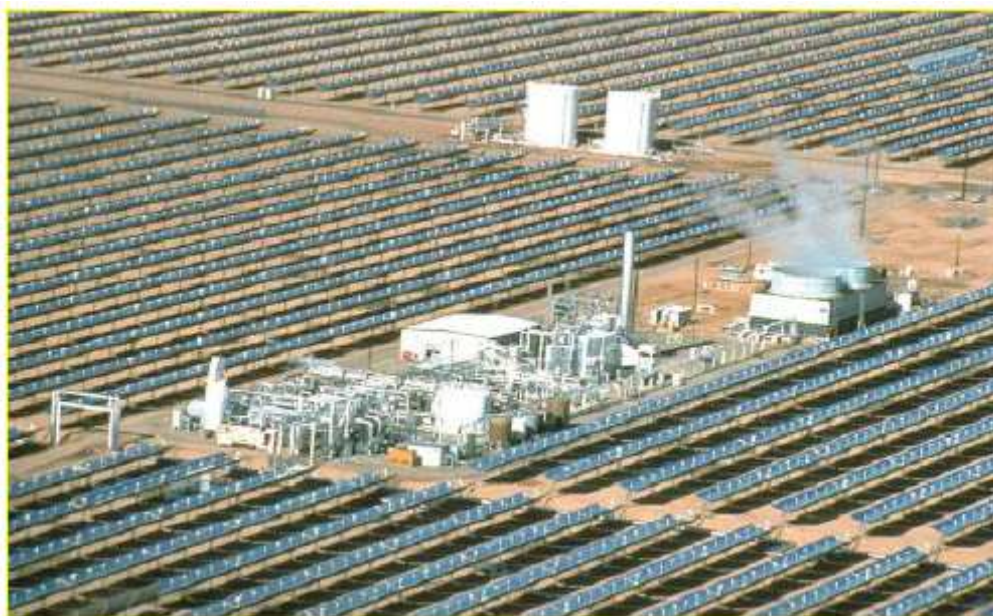
Figure 10: Centrale solaire thermodynamique (Source: ADEME)
